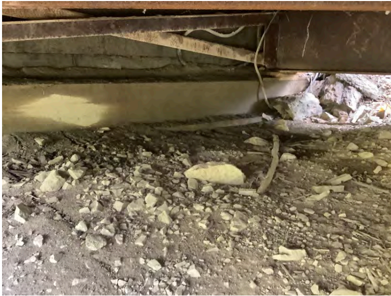
Left Bank Abutment when facing downstream
