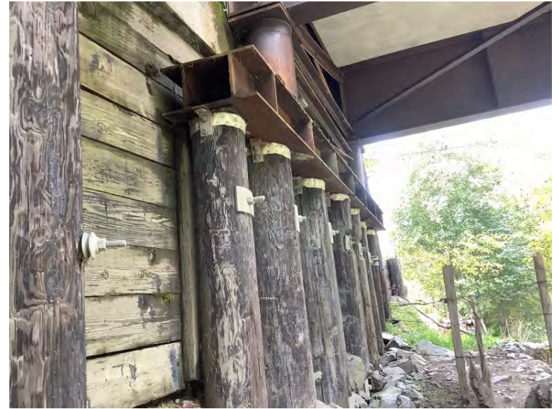
Left Bank Abutment when facing downstream
